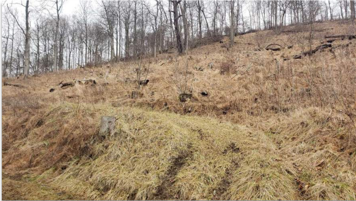
PHOTO 3: Topsoil slide along property
